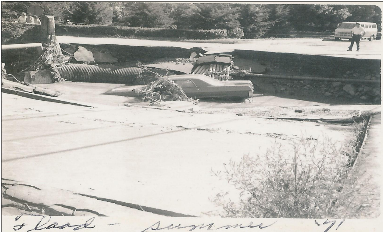
Figure 14. Damage from Hurricane Doria to a road adjacent to the Peckman River (1971).
