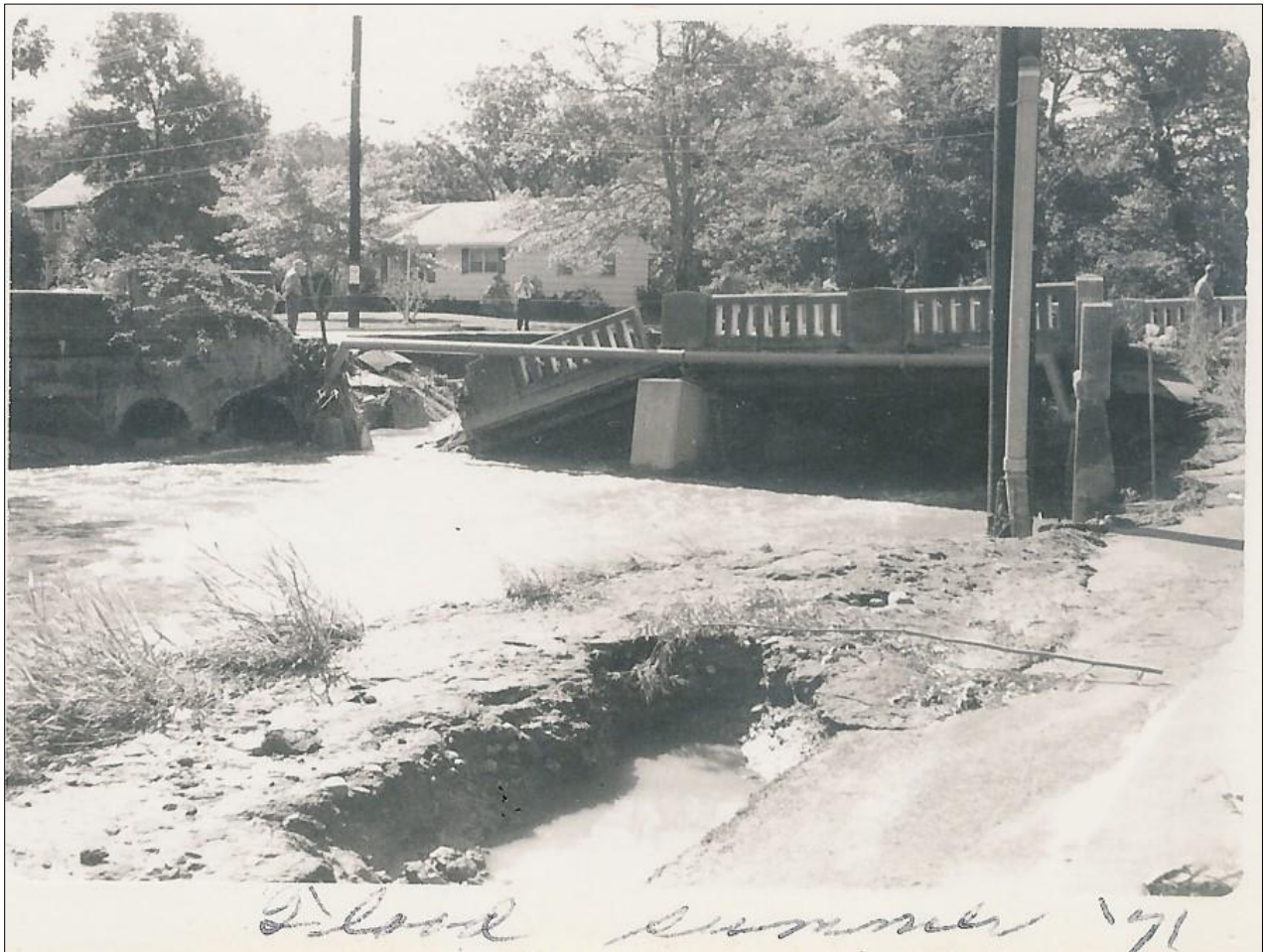
Figure 20. Damage from Hurricane Doria to a bridge abutment & road along the Peckman River (1971).
