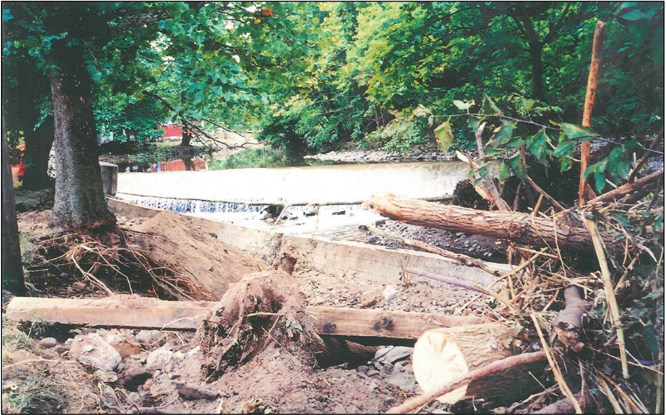
Woody debris and erosion left in the aftermath of Hurricane Floyd (September 1999).
