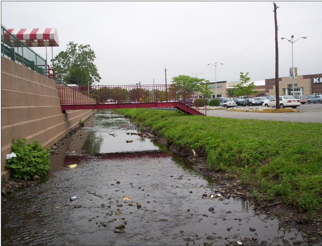
Figure 30. Pedestrian Bridge over Great Notch Brook at the commercial retail property, Woodland Park, New Jersey (2017).
