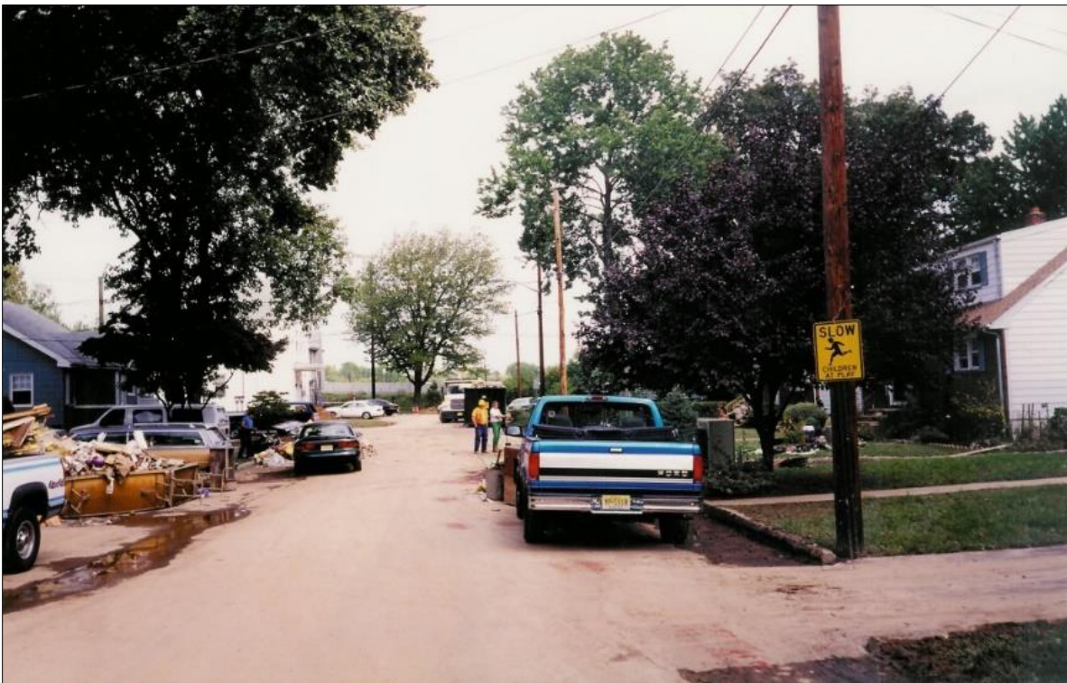
Figure 12. Repairs being performed on a property due to Peckman River flood damage from Hurricane Floyd (1999).
