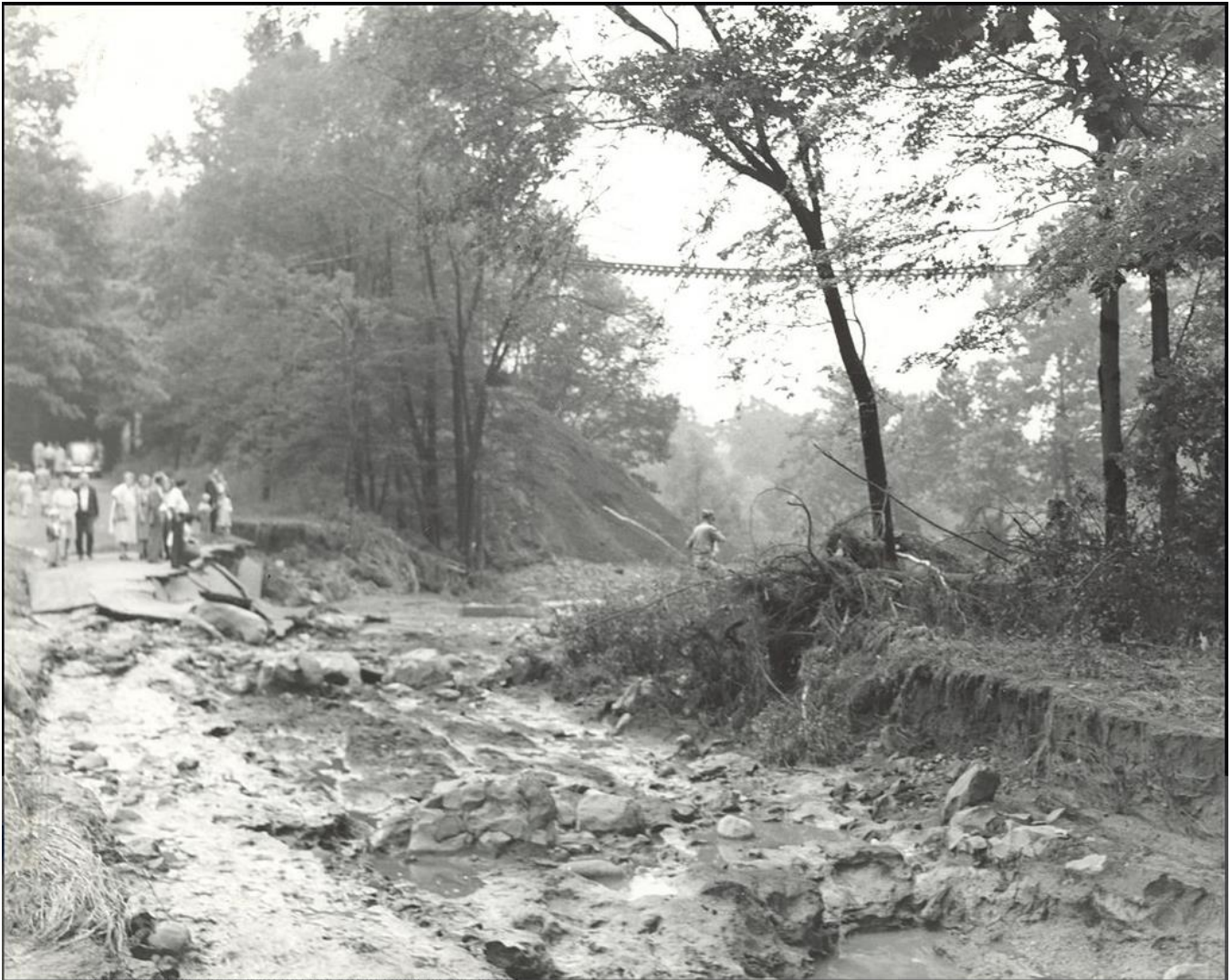
Figure 18. Erie Railroad tracks suspended in the air after the Peckman River flood of July 1945 washed away the earth supporting the bridge for the tracks. Courtesy of the Little Falls Historical Society. Photographed July 22, 1945.
