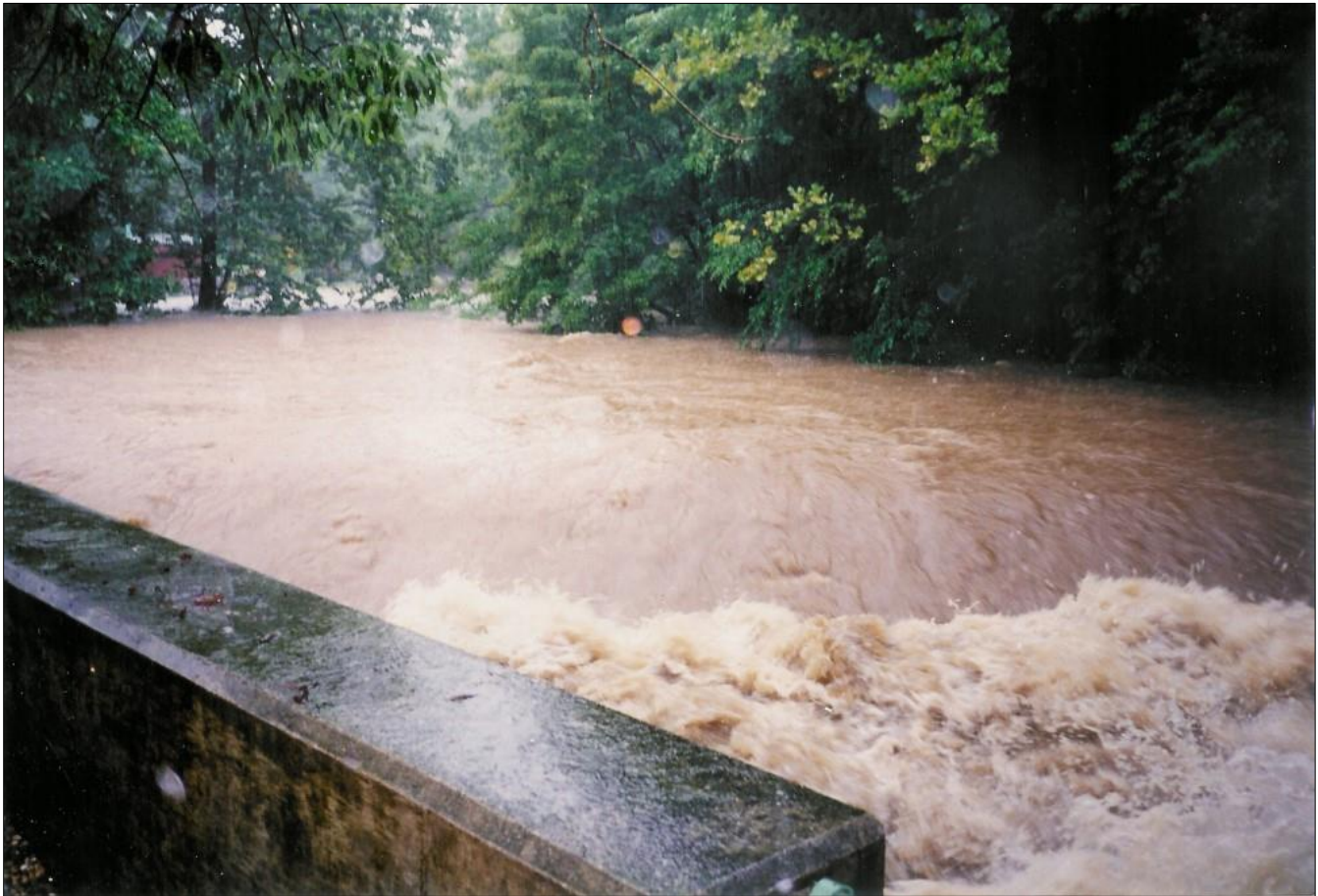
Figure 21. High flows and water levels due to Hurricane Floyd at a bridge abutment along the Peckman River (1999).
