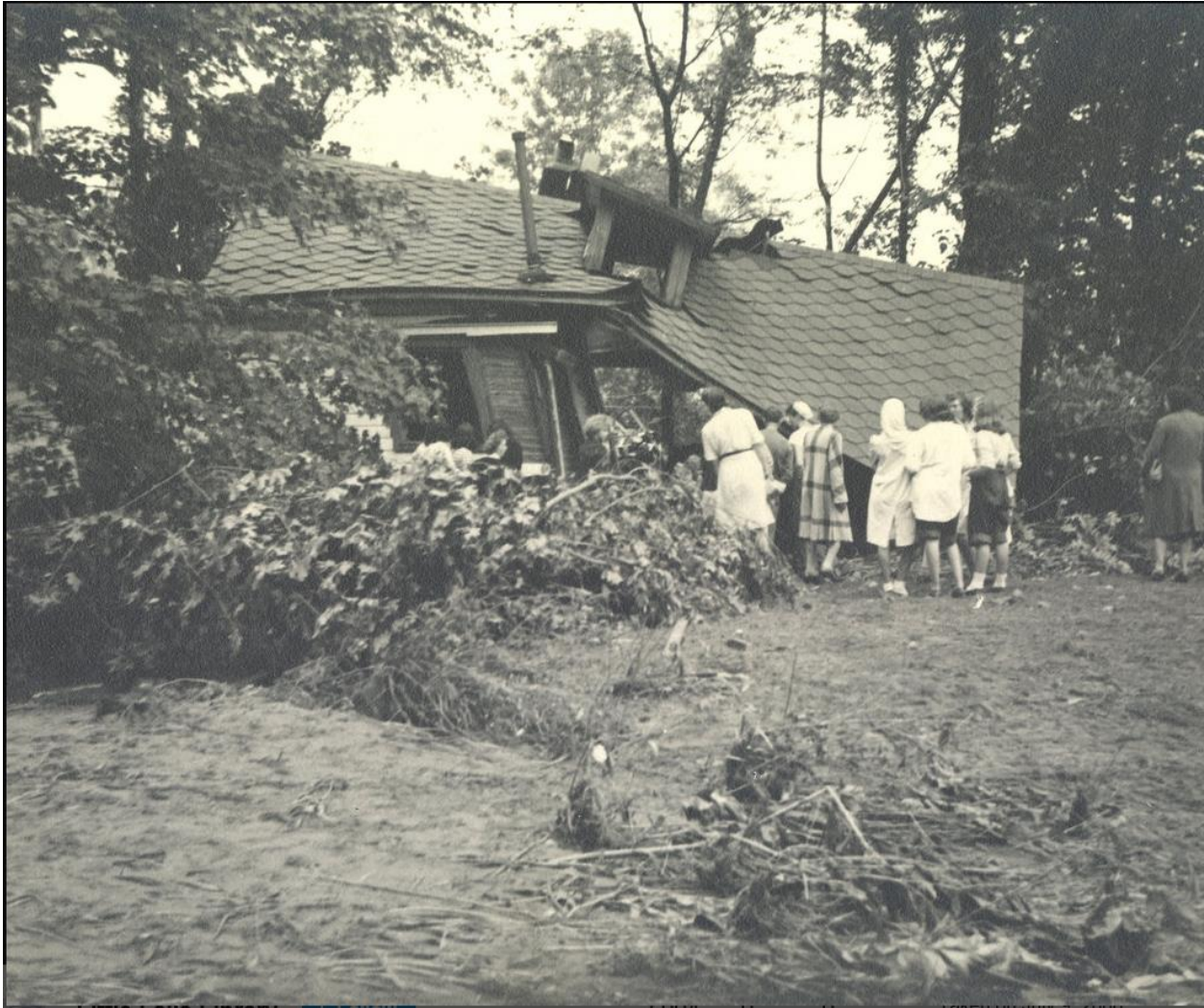
Figure 19. The Riker family house on Cedar Grove Road in Little Falls, NJ after it had been destroyed by the Peckman River flood of 1945. The house was split down the middle and collapsed. The house was washed from its foundation and collapsed, killing a woman who lived there. Courtesy of the Little Falls Historical Society. Photographed July 22, 1945.
